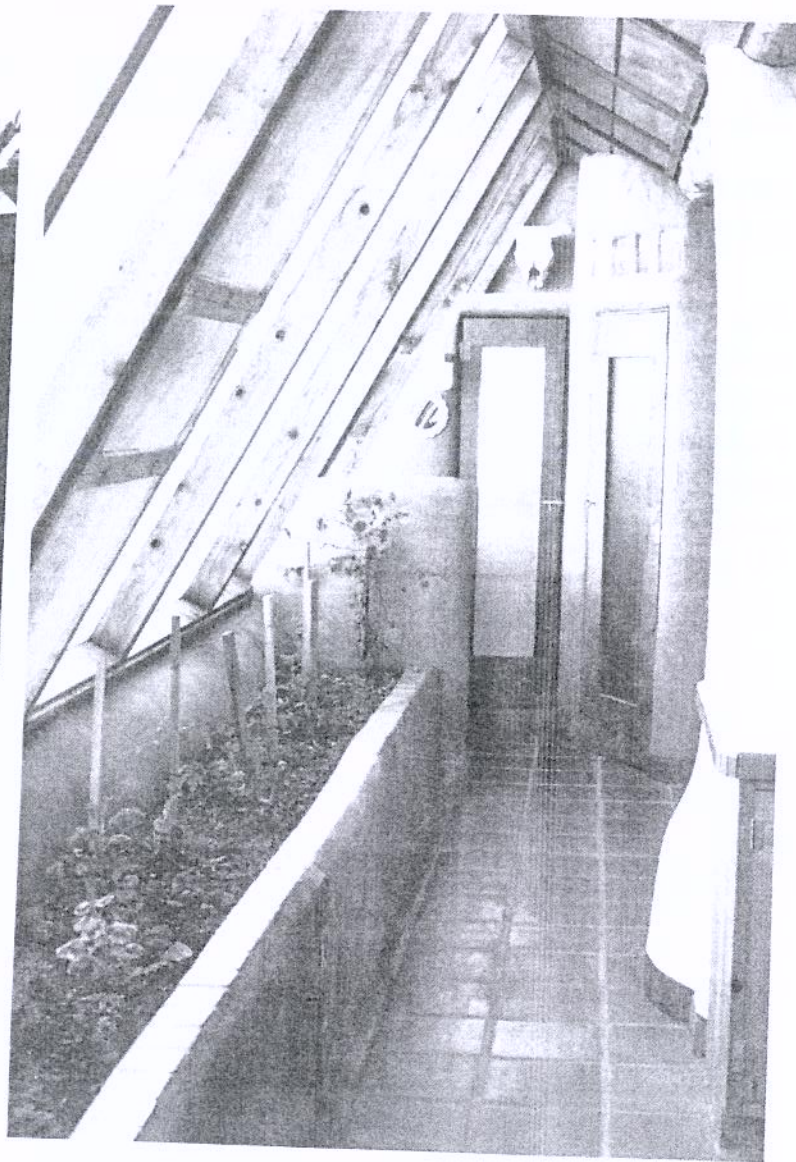
Finished Greenhouse - interior.
