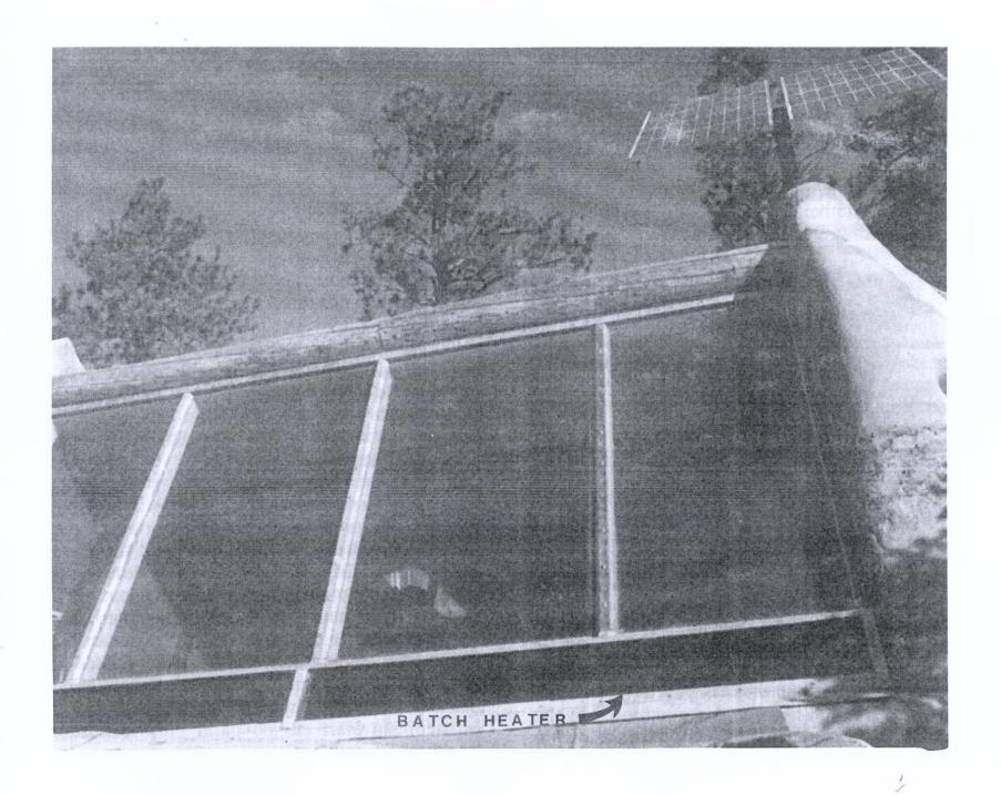
Water is pumped into the tank from below until the tank overflows (outside or into a planter). The water is then heated by the sun and allowed to flow back down the same pipe that filled it and into the hot water lines. This involves some simple valving to close off the supply of cold water to fill the tank and open the hot water (gravity fed) to the hot water taps.
