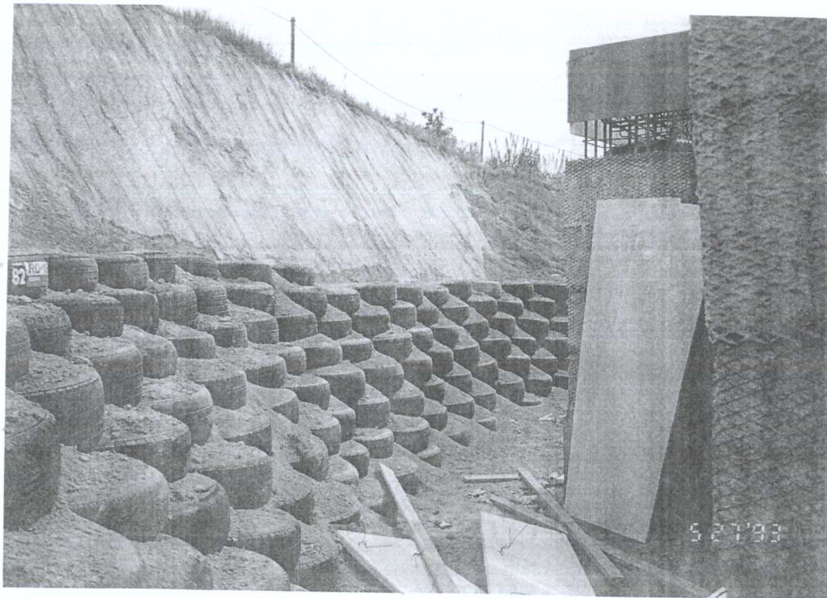
TIRE RETAINING WALL BEHIND EARTHSHIP IN JAPAN.
