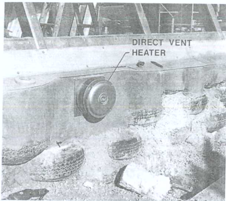
A direct vent heater through the front face tire wall shown above.
