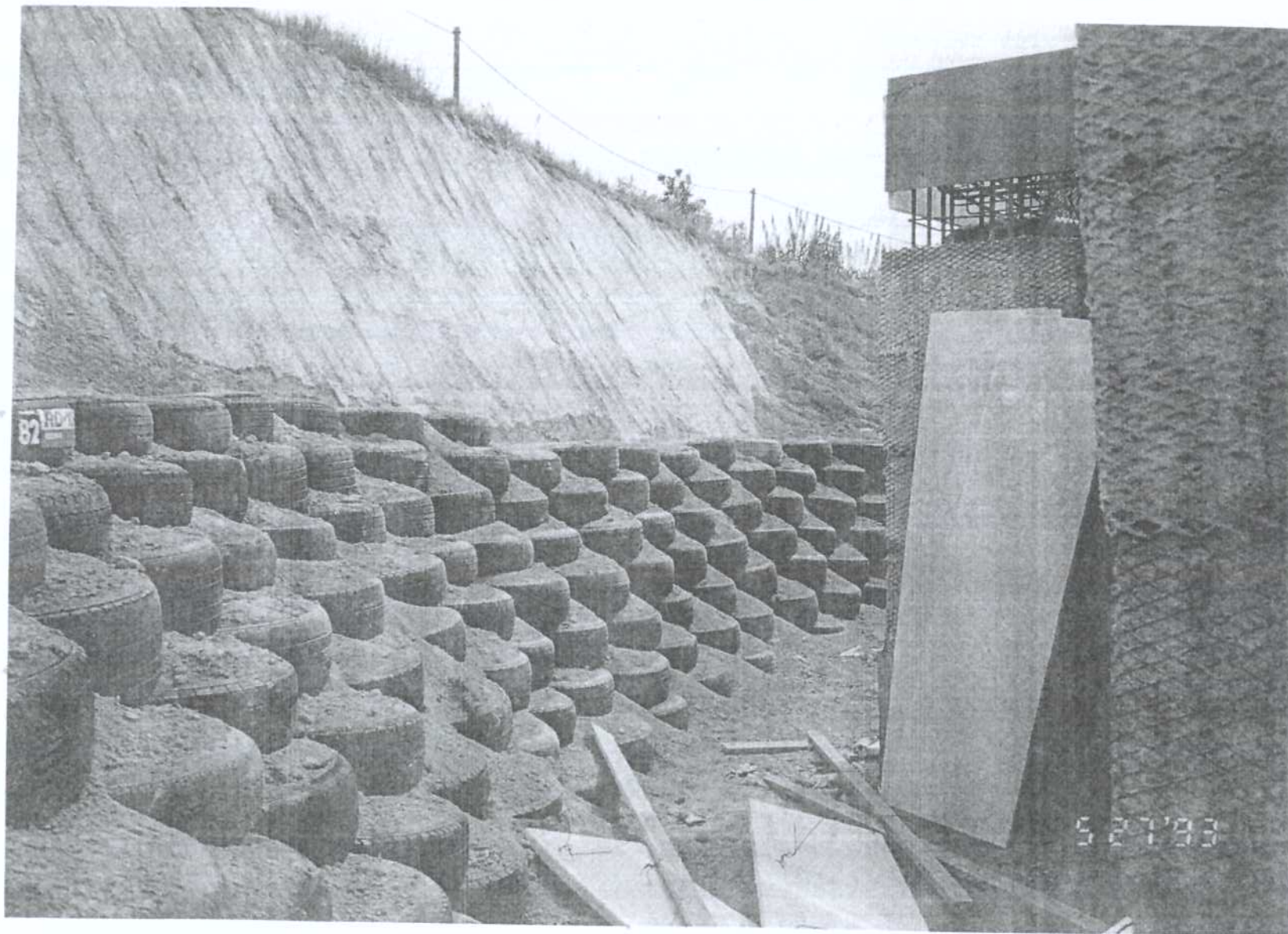
TIRE RETAINING WALL BEHIND EARTHSHIP IN JAPAN.
